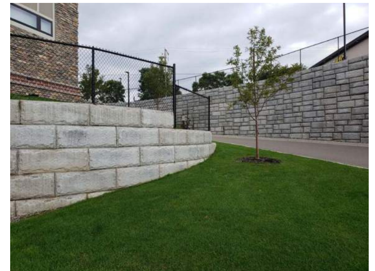
SCALE: LARGE SCALE STONES ON THE BOTTOM OF WALL SMALL SCALE, VARIOUS PATTERN ON TOP OF WALL
