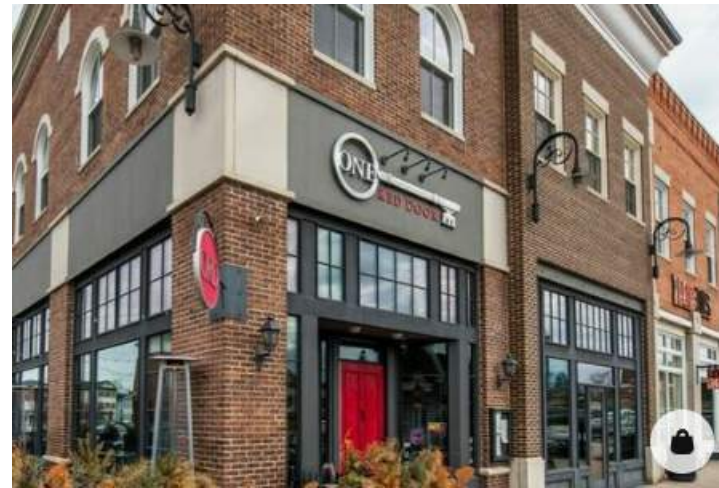
DEFINED BASE: BELT COURSE, STONE PILASTERS STORE FRONT VIBE
